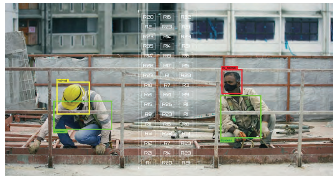
Artificial intelligence (AI) and machine learning technologies will be applied to video feeds captured on drones and robotic systems to automatically identify safety lapses in real time.
