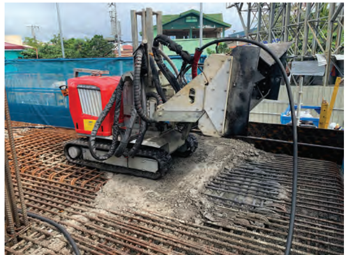
ABOVE AND BELOW: With the ability to complete concrete removal tasks up to 25 times faster than a hand lance, the Aquajet Aqua Cutter provided the necessary solution to keep the project on schedule.
