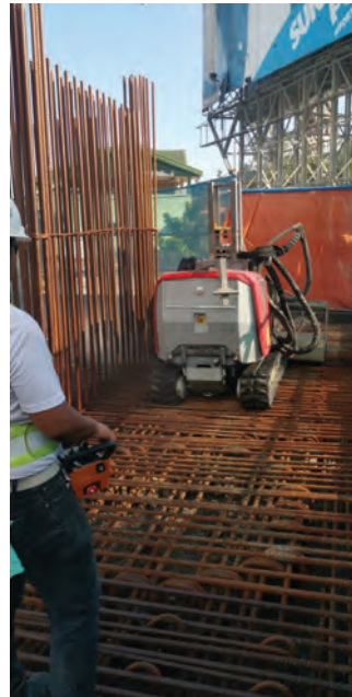
FAR LEFT: The uneven, muddy terrain at the jobsite presented no problems for the self-propelled Aqua Cutter hydrodemolition robot. This minimised necessary site preparations and helped accelerate repairs.
