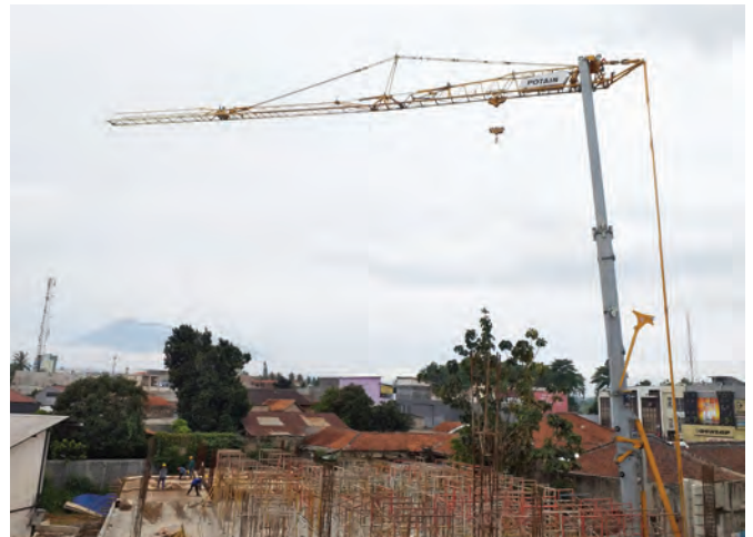
The Potain Hup 32-27 self-erecting crane on a project site.
