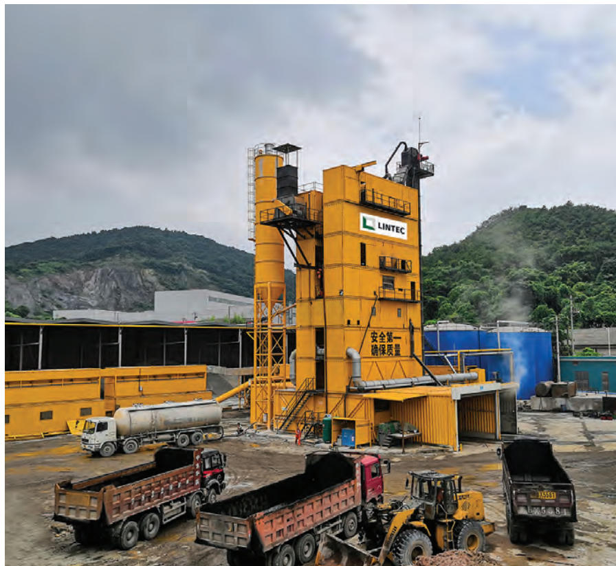
The Lintec CSM4000HS20-SE asphalt plant has been used to deliver over 3,000 t of asphalt per day. Materials from the plant are delivered to a host of the contractor's regional projects, including the phase four expansion project of Ningbo Lishe International Airport as well as numerous surrounding highways.
